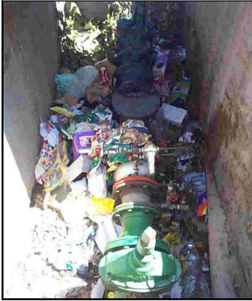
**Figure 4.11: Valve Chamber Requiring Cleaning and Securing**
