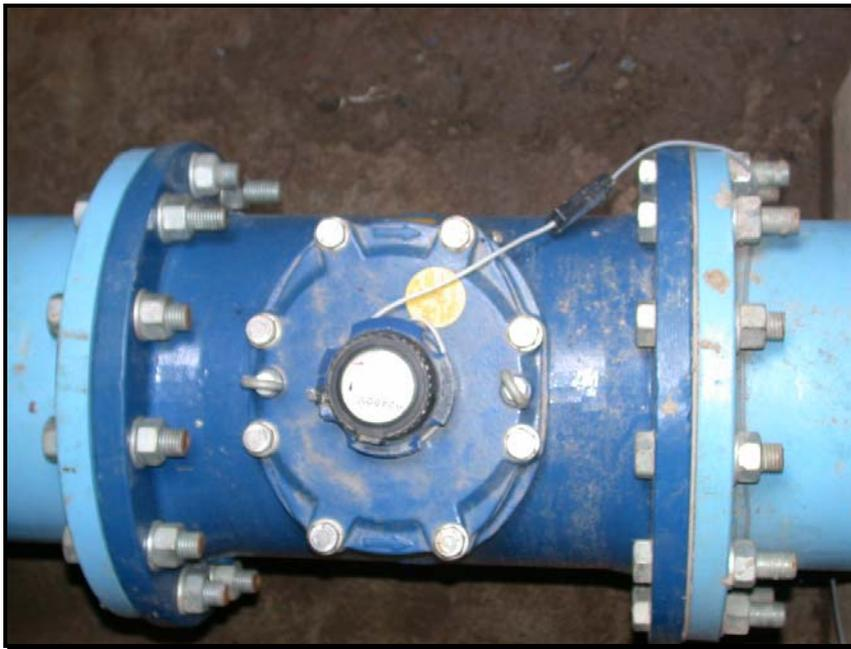
**Figure 4.16: Typical Turbine Flow Meter**
