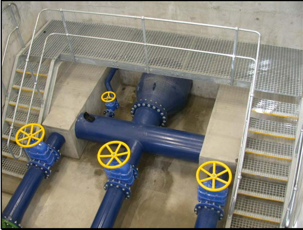
**Figure 3.10: Typical Isolating Valves (four gate valves)**
