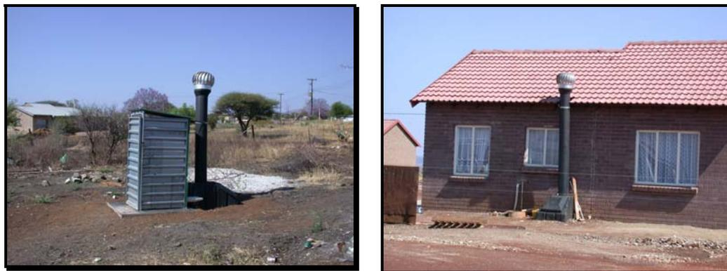
**Figure 5.3: Waterless toilet installations (Courtesy WRP (Pty) Ltd)**
