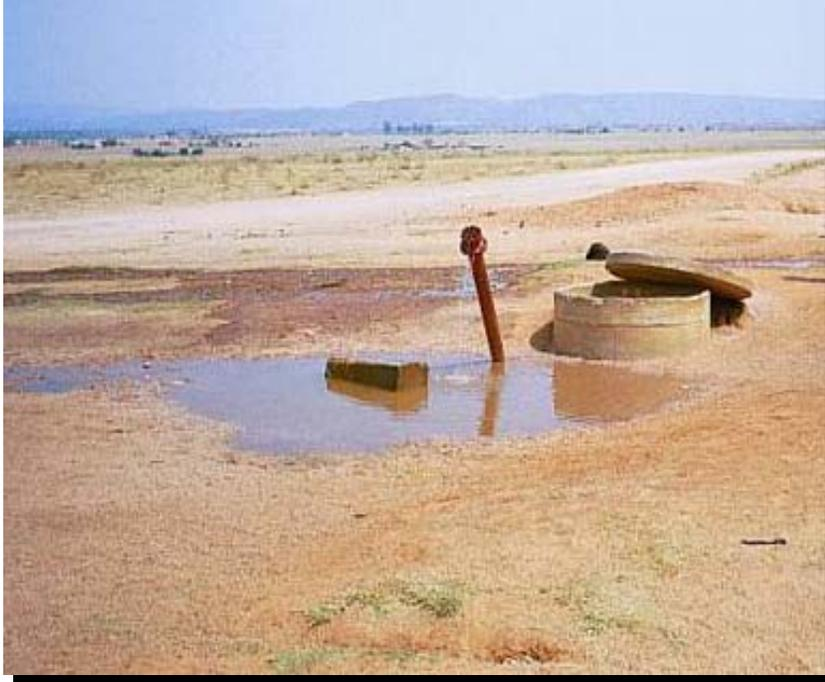
**Figure 3.14: Leaking Scour Valve (vandalised to provide for stock-watering)**
