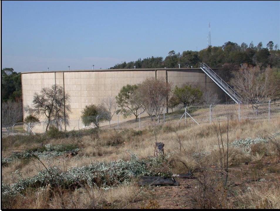
**Figure 3.7: Typical Bulk Storage Reservoir (24 MI)**
