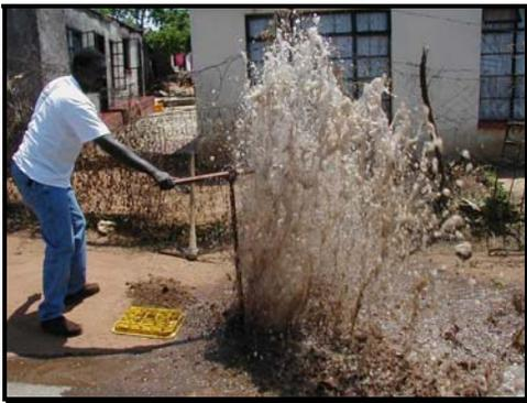
**Figure 3.8: Mains Flushing to Remove Silt from Pipeline**
