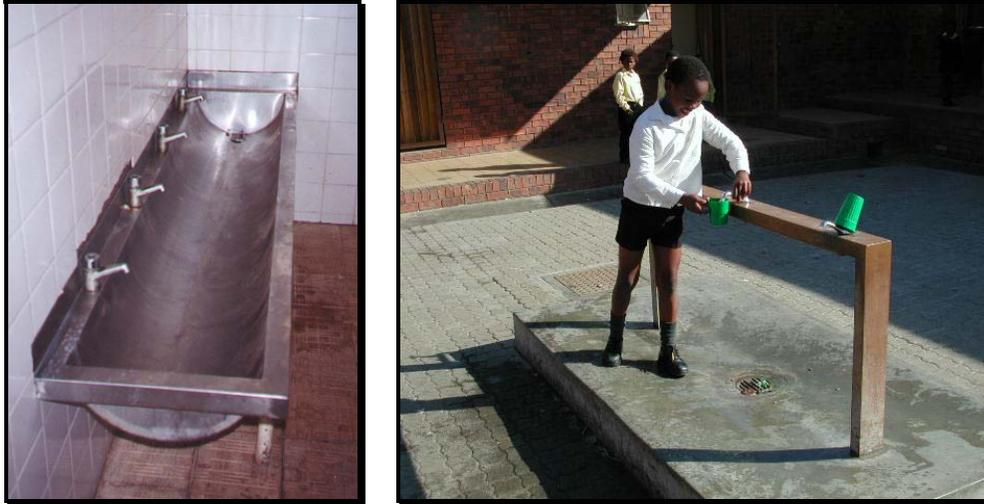
**Figure 5.11: Self-Closing Taps installed at a school (Courtesy Ayanda Consulting)**
