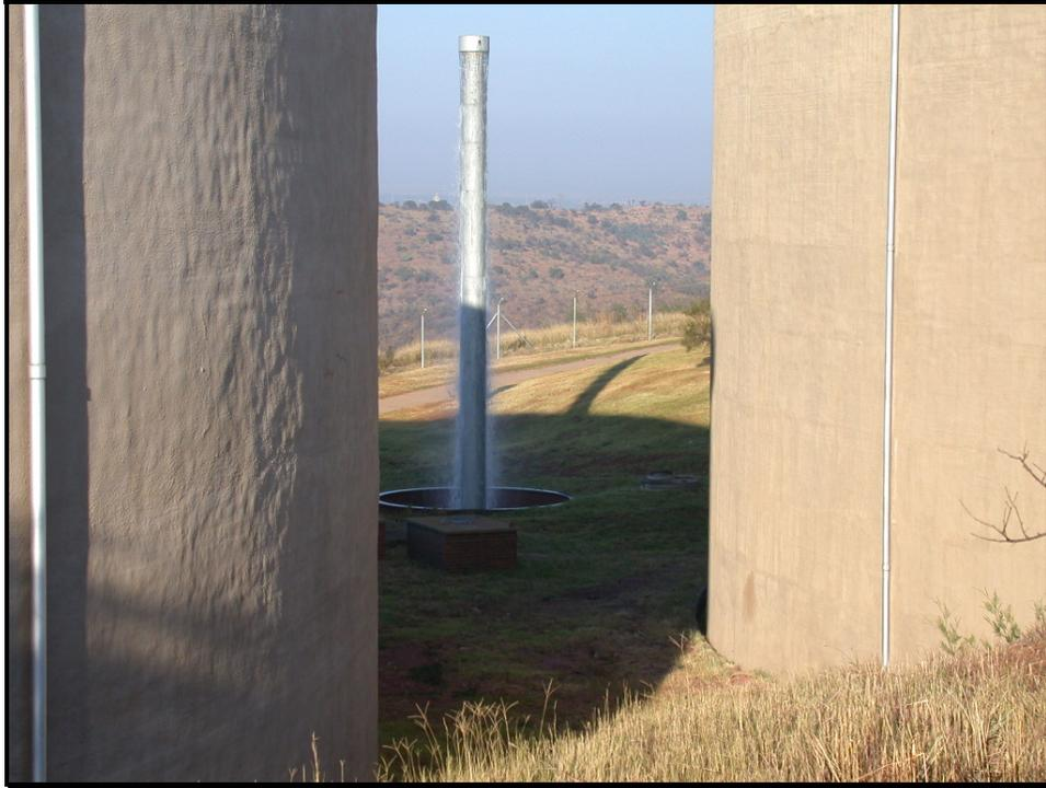
**Figure 3.8: Overflow from a Bulk Storage Reservoir**
