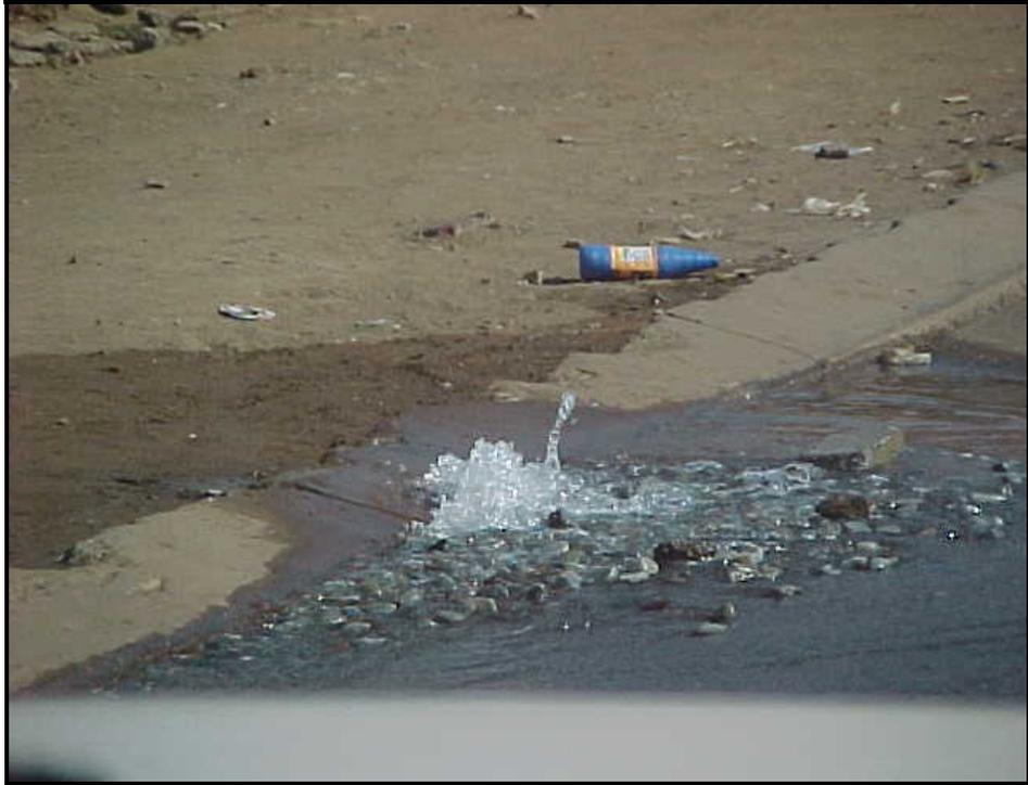
**Figure 2.4: Typical Connection Pipe Burst**
