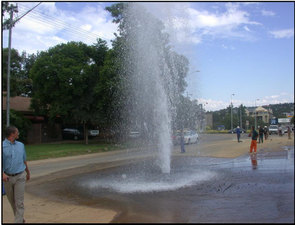
**Figure 2.3: Typical Mains Burst**
