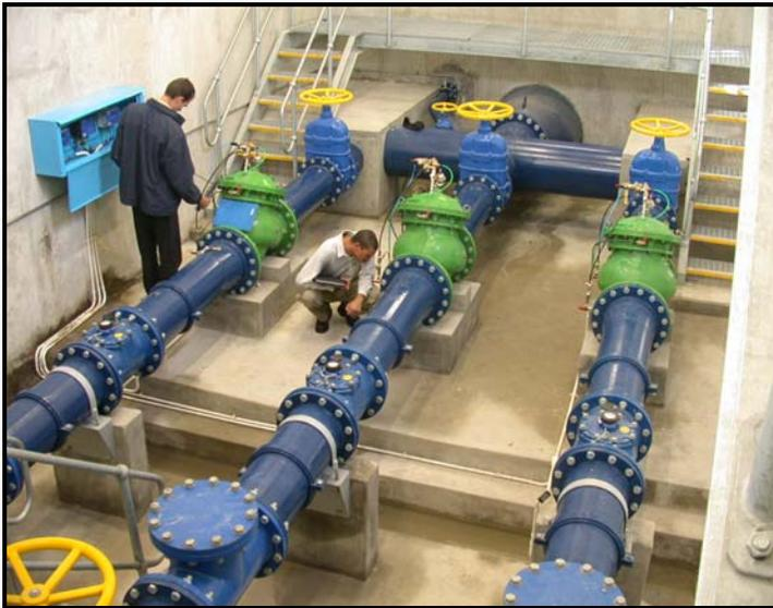
Figure F3: Internal View of a Portion of the 1065 mm diameter Chamber
