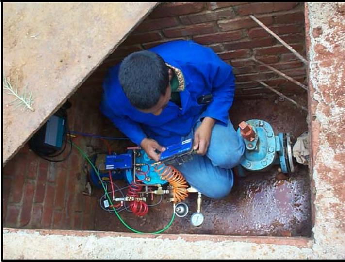
**Figure 4.18: Installation of Loggers** (courtesy Pressure Management Systems)
