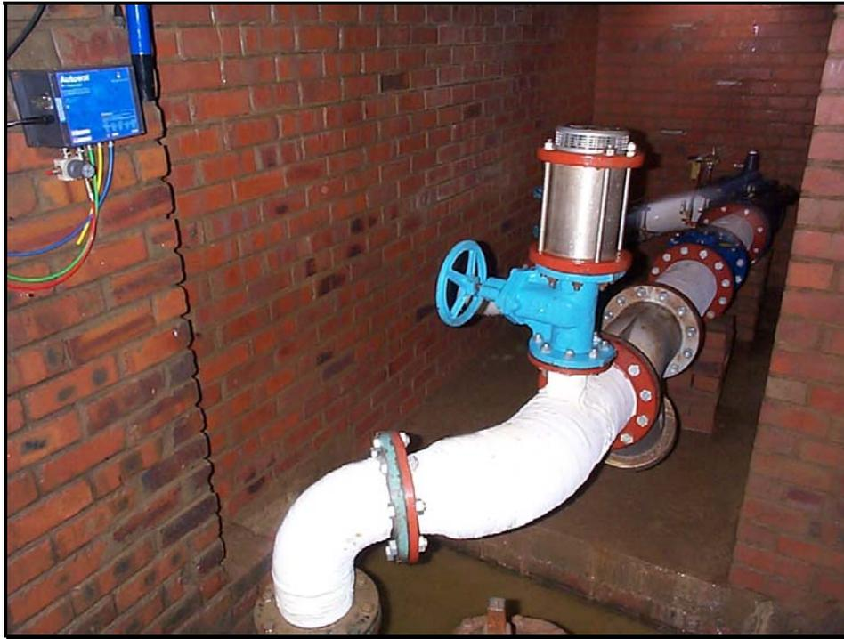
**Figure 3.13: Typical Air Valve (Silver/Red) on Top of Isolating Valve (Blue)**
