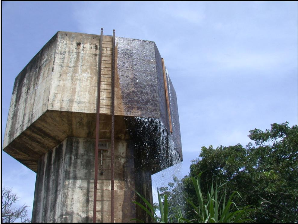
**Figure 2.7: Example of a Reservoir Overflow**
