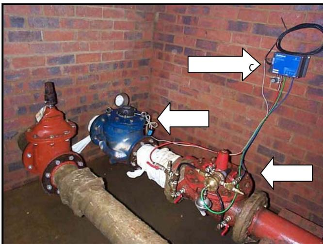
**Figure 4.8: Typical Flow-Modulated PRV Installation**
