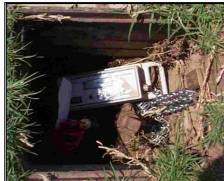
**Figure 4.13: Pressure Logger Installation on a House Connection and Fire Hydrant**
