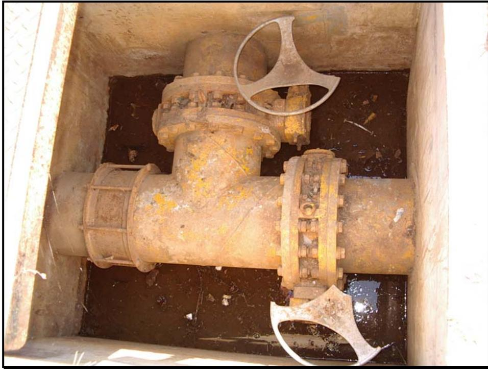
**Figure 3.9: Leaking butterfly valves with broken spindle handles**
